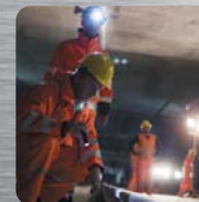
Railway works and repair
