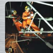
Electric power & Communication rush repairs
