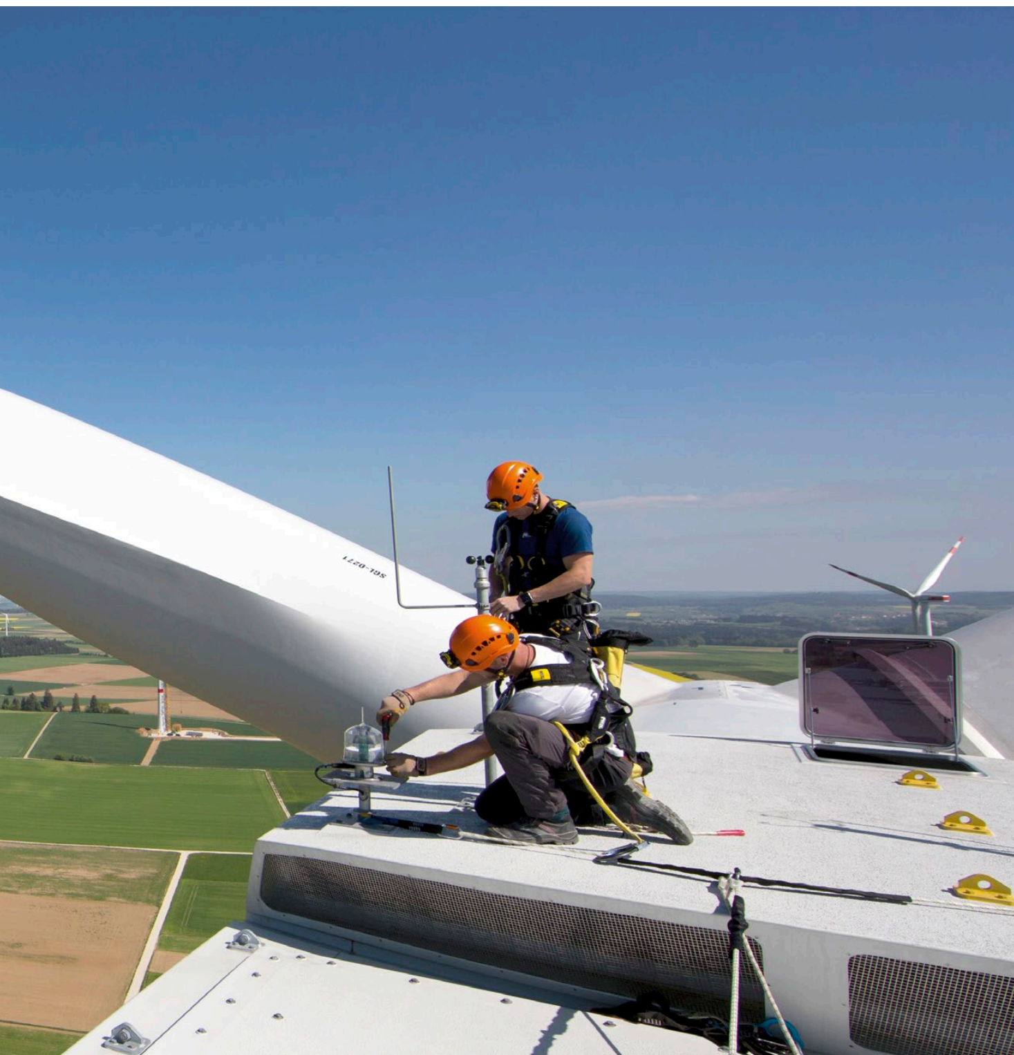
Maintenance on a wind meter and beacon light at the top of a modern wind turbine. Deining, Deutschland. © Petzl / Lafouche / Max Bögl
