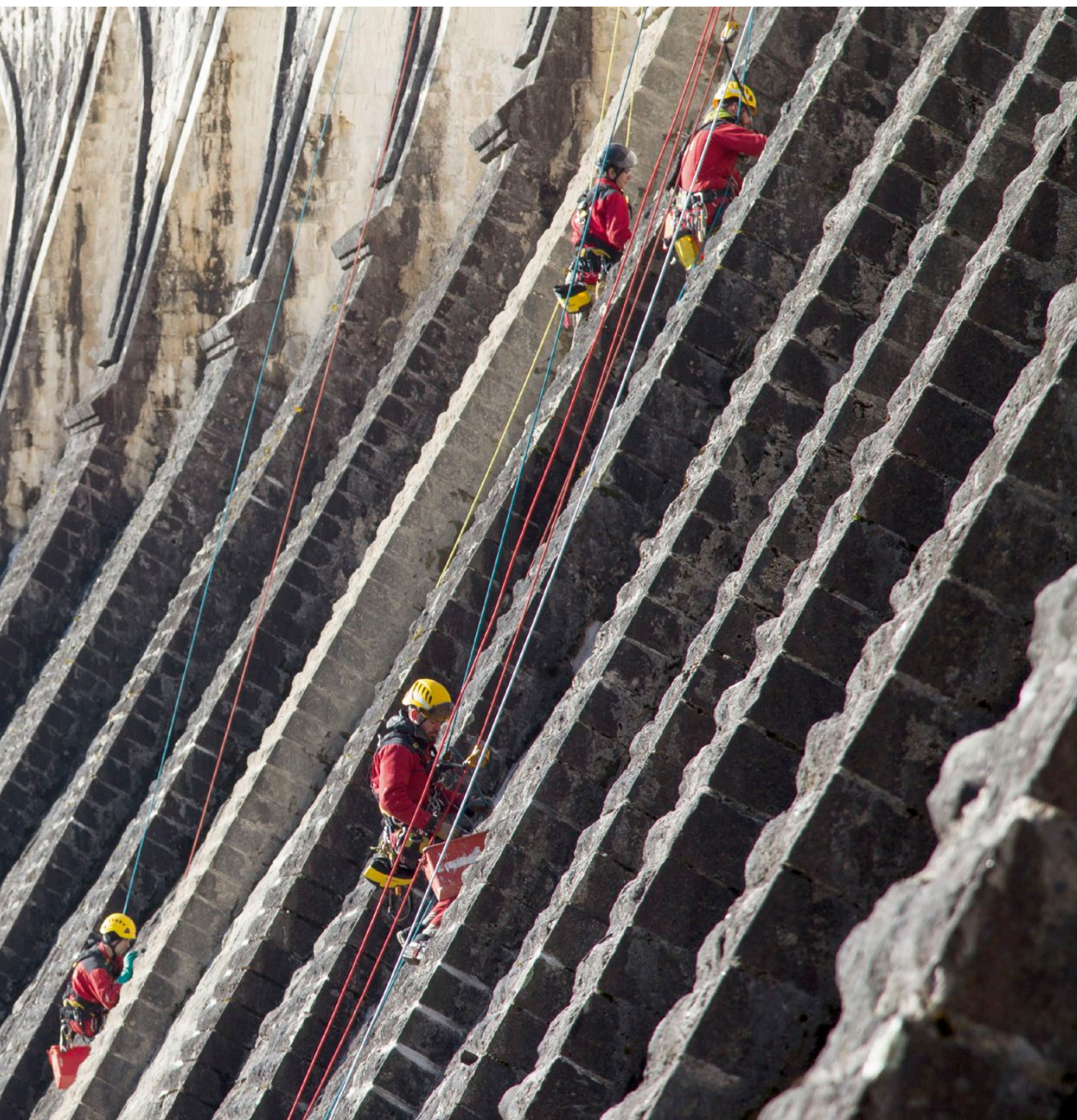
Reworking the masonry on the Chartrain Dam maintained by the Roannaise de l'eau in Loire, France. © Petzl / vuedici.org / L. Moretton
